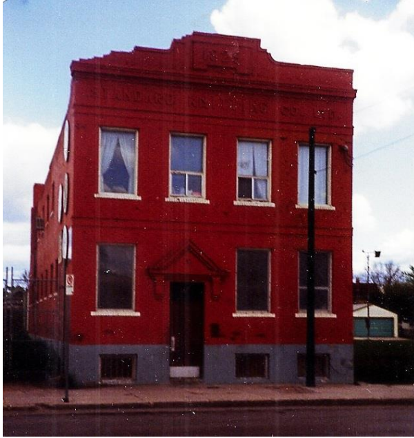
Standard Knitting building, repainted, in its second incarnation as a community centre, circa 1975. The Halparin family home occupied the empty lot to the right.
